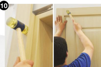
10 Double-side adjusted cornice are cut according to the measurement and fitted by using a plastic hammer.
