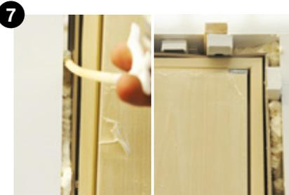
7 Apply polyurethane foam in the gap between the frame and wall. After drying, remove the foam residues.
