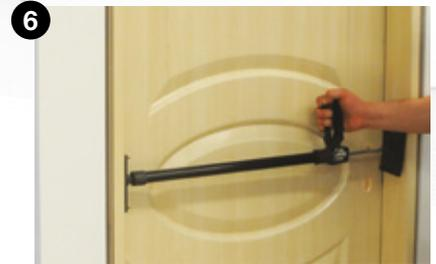
6 Adjust the internal measurement between sash and frame as 3.5 mm by using an adjuster. Frame - Sash balance should be checked again.
