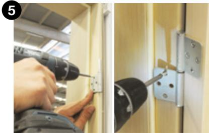
5 Upper hinge center is screwed to the frame as 254 mm from above.
