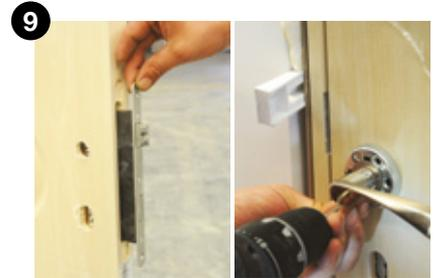
9 Lock and handle suitable for the leaf are fitted by screwing them.
