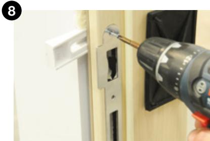
8 Lock is screwed to the drilled area in the frame.
